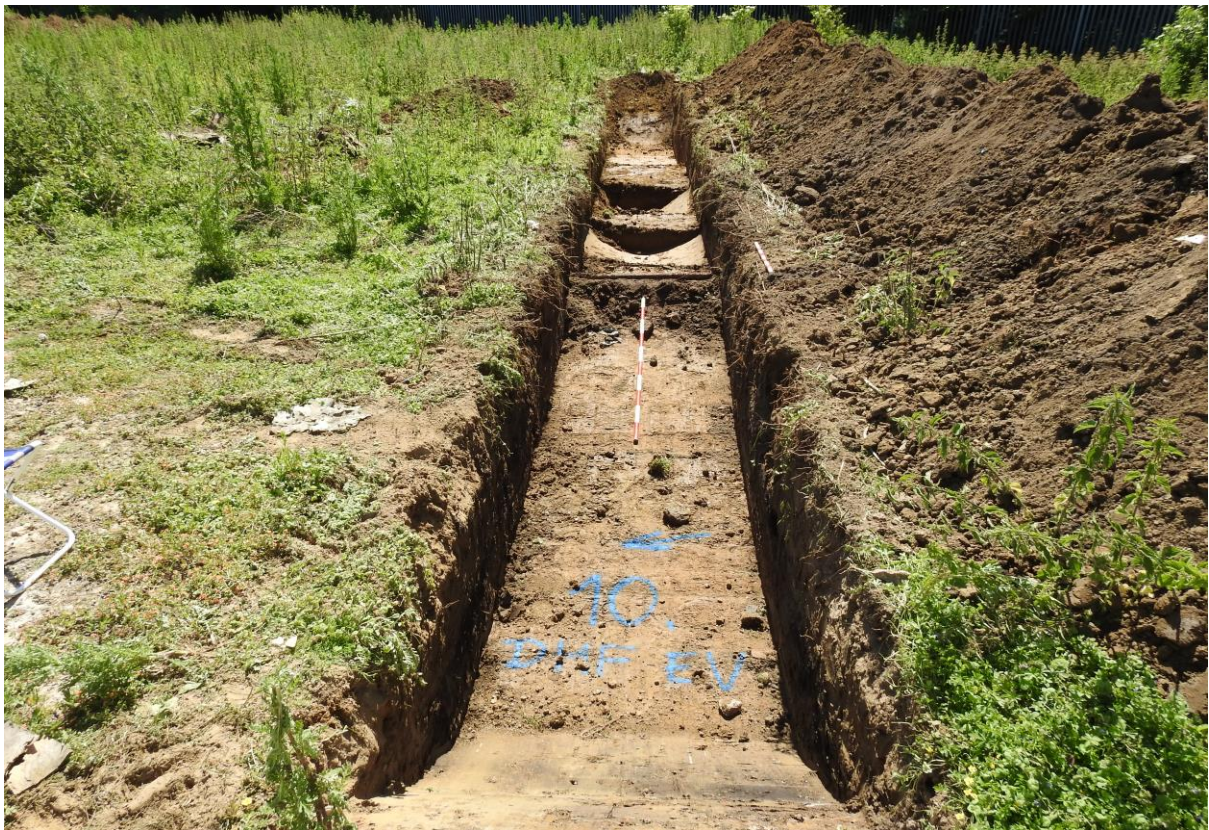
Plate 8: Trench 10 viewing from west with one- and two-metre scales.
